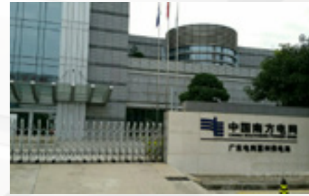
Huizhou Power Supply Bureau of Guangdong Power Grid Co. Ltd
