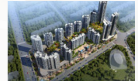
Jiangzhou Huafu, Jiujiang City, Jiangxi Province
