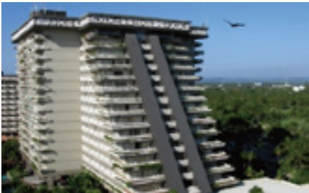
Mexico Commercial Building
