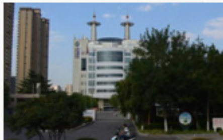
China Mobile Communications Group, Jiaozuo branch, Henan
