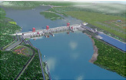
Datengxia Water Conservancy Guangxi Province
