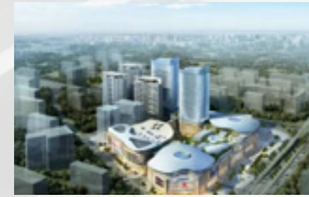
Wangfujing Department Store, Foshan City, Guangdong Province
