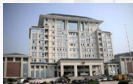
Qujiang Public Security Bureau, Shaoguan, Guangdong Province
