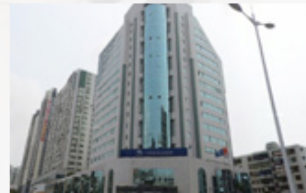
Zhanjiang Power Supply Bureau of Guangdong Power Grid Co. Ltd.
